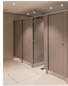
Example image: WC cubicles
